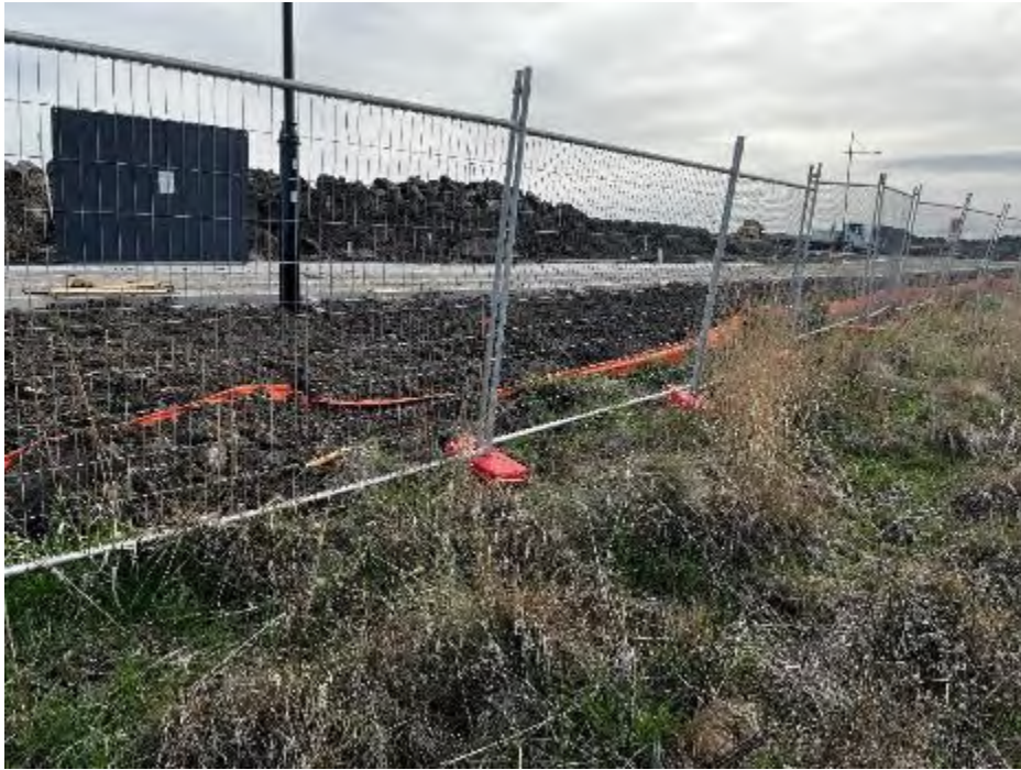
Photo 8: Collapsed and damaged sediment fencing.
