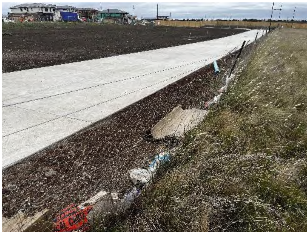
Photo 25: No sediment fencing adjacent areas of construction and earthworks.
