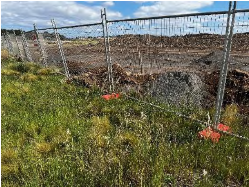
Photo 9: Sediment fencing not present around areas of earthworks
