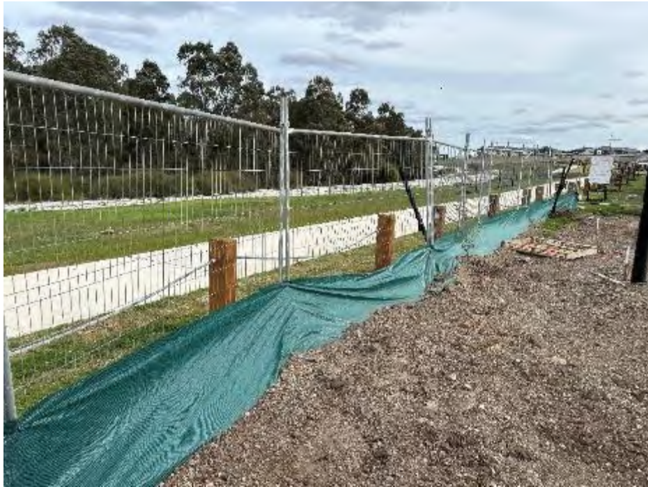
Photo 10: repaired sediment fencing. Provided by DFC Oct 2024.
