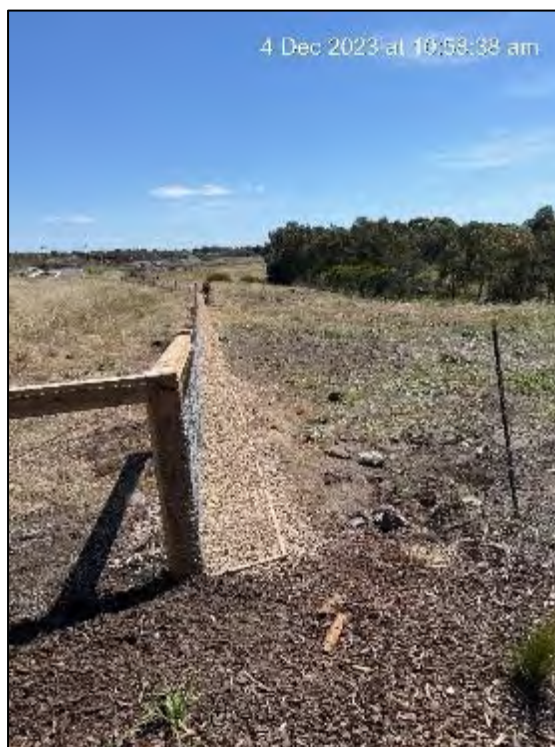
Photo 20: Permanent fencing upgrade around grassland reserve as part of stage 33.
