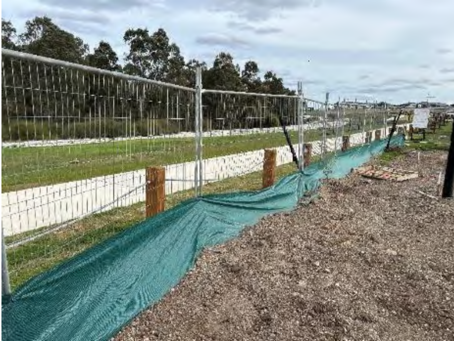
Photo 9: repaired sediment fencing. Provided by DFC Oct 2024.
