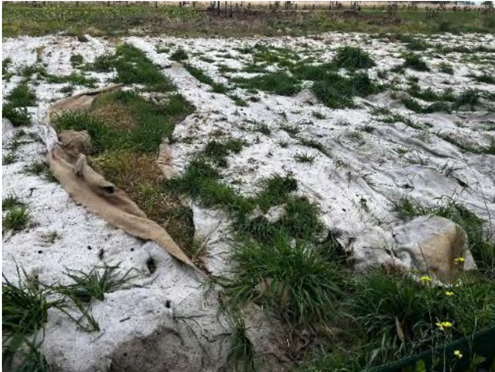
Photo 3: Evidence of degraded revegetation works along the GGFMB in the east of the study area.
