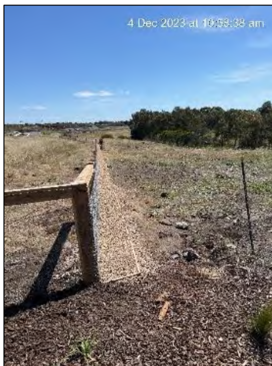
Photo 15: Permanent fencing upgrade around grassland reserve as part of stage 33.
