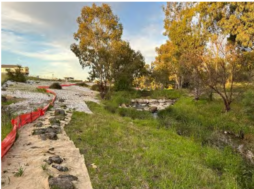
Photo 1: Revegetation works in the south-east portion of the GGFMB
