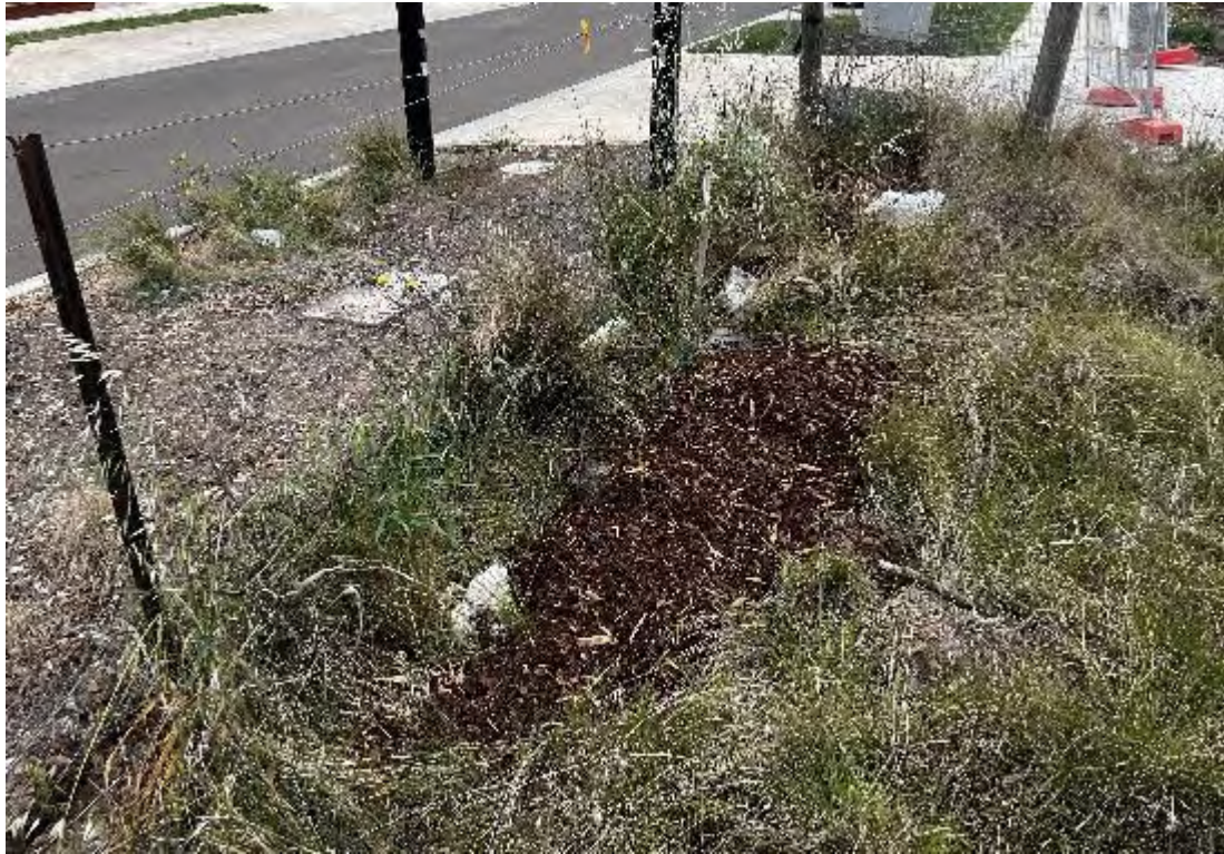
Photo 16: Mulch pile along roadside fencing, with tampered fencing.
