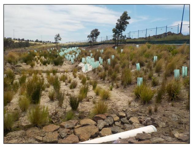
Photo 2: Revegetation works associated with a drainage swale
